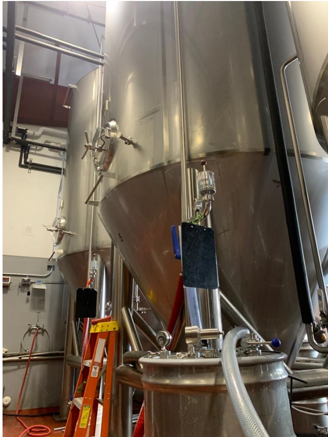
Focus Capture CO2 off Fermentation Tanks
